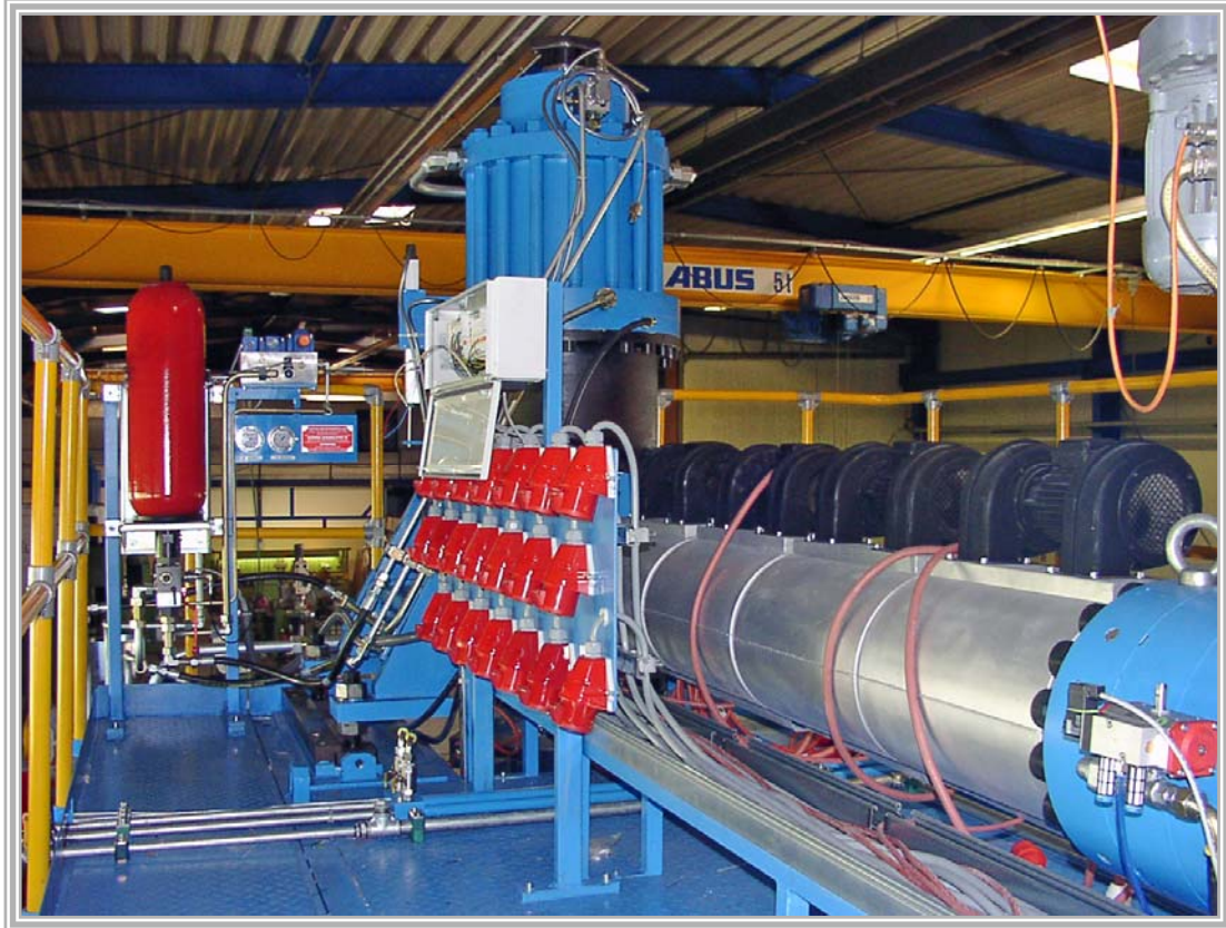
B-750: view of extruder platform
